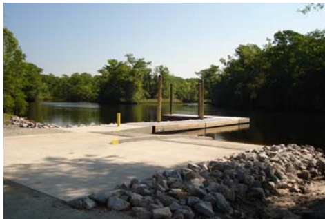
New ramps and floating dock at Pitch Landing.
